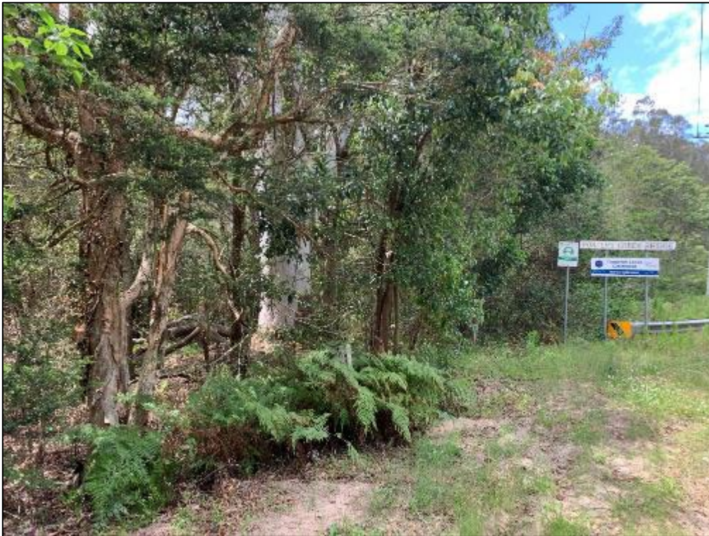
ABOVE: Porters Creek Bridge on northern side - Noted Landcare site adjacent
